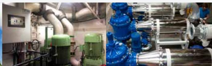
The OptiSave™ system automatically adjusts the speed of the vessels cooling system pumps to the actual cooling need, which can lead to significant annual energy savings. This is well documented by the more than 100 OptiSave™ systems sold by DESMI to date.
